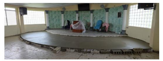
small task as all the sand, gravel and concrete had to be wheeled in one wheelbarrow at a time. The concrete was mixed on the ground by hand, loaded in wheelbarrows by shovel and carried
